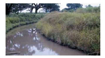
A permanent irrigation canal or lateral constructed to move water from the source of supply to one or more farms. The conservation objectives are to prevent erosion or degradation of water quality or damage to land, to make proper water use possible and to move water efficiently.
