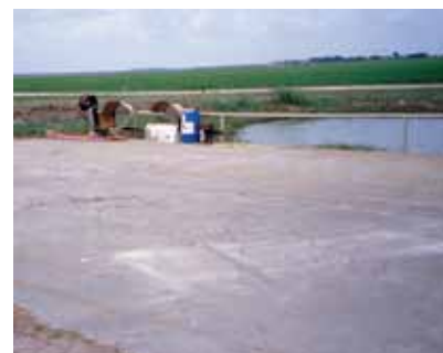
Wash pad with collection pond
