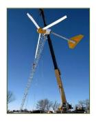
turbine powers groundwater circulation wells used for air stripping and ultraviolet (UV) treatment. The system reduces consumption of utility electricity by 26% during grid intertie mode but can also operate off-grid when needed. Over 15 years, the electricity savings could exceed \$40,000. Estimates at the time of wind turbine installation (2003) suggested that a similarly sized system operating fully off-grid would cost approximately \$45,000.
