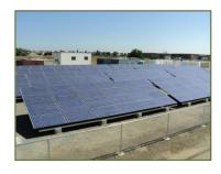
building. The PV system now meets 100% of the remediation system's annual energy demand, which encompasses operation of 16 wells that extract groundwater for treatment in granular activated carbon vessels.
