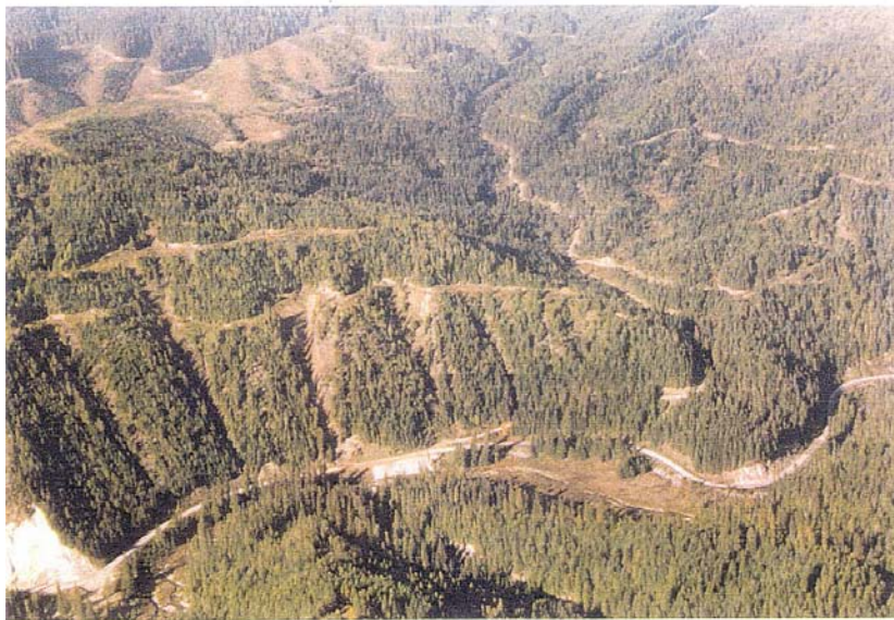
Figure 1. Road-initiated debris flows in inner gorges, main stem Beaver Creek, North Fork Clearwater River.
