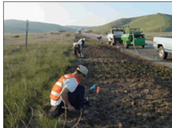
Another CalTrans site along the roadside that is being planted with native grasses.
