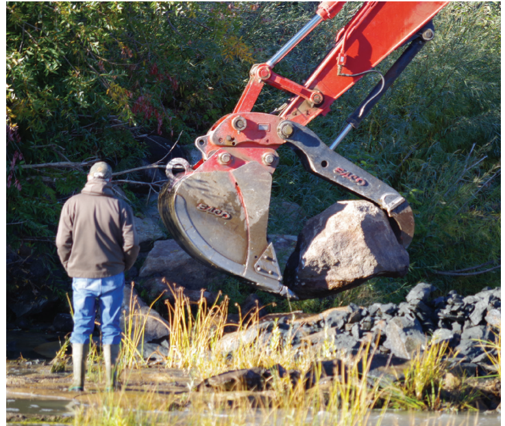
Hickey directs a contractor installing rock bars to protect against future floods.
