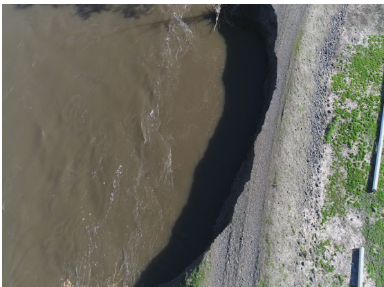
Flood waters washed away a levee road on the Weiser River. Photo credit Snake River Horizons, 2017.
