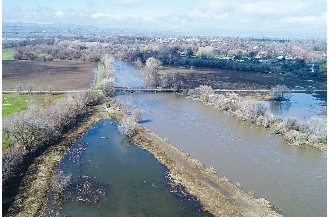
Aerial footage captured by Snake River Horizons shows the flooding, damaged sediment-retention ponds, and levees by Twin Bridges.
