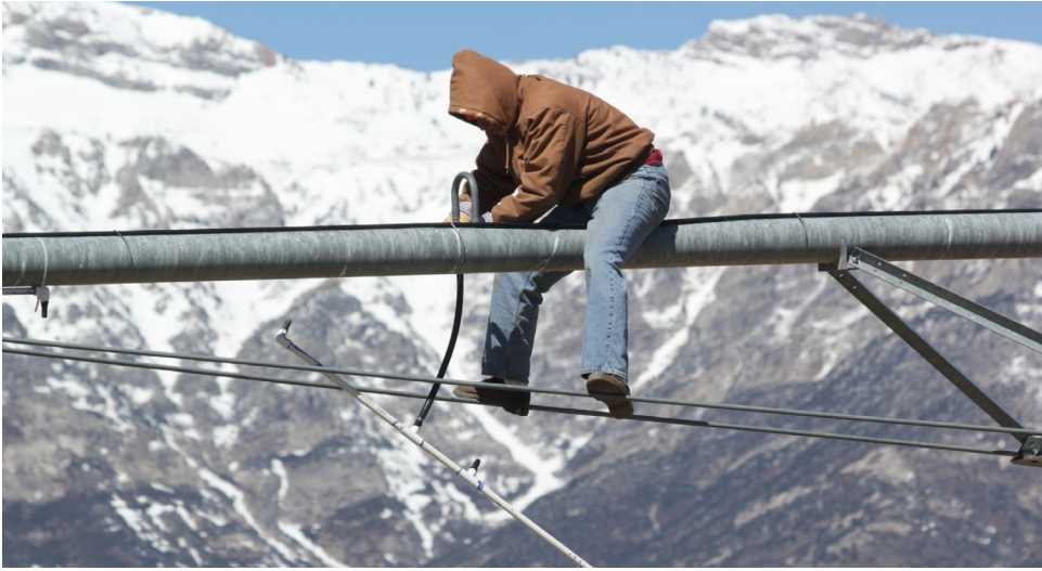
Assembling LESA can be precarious.
