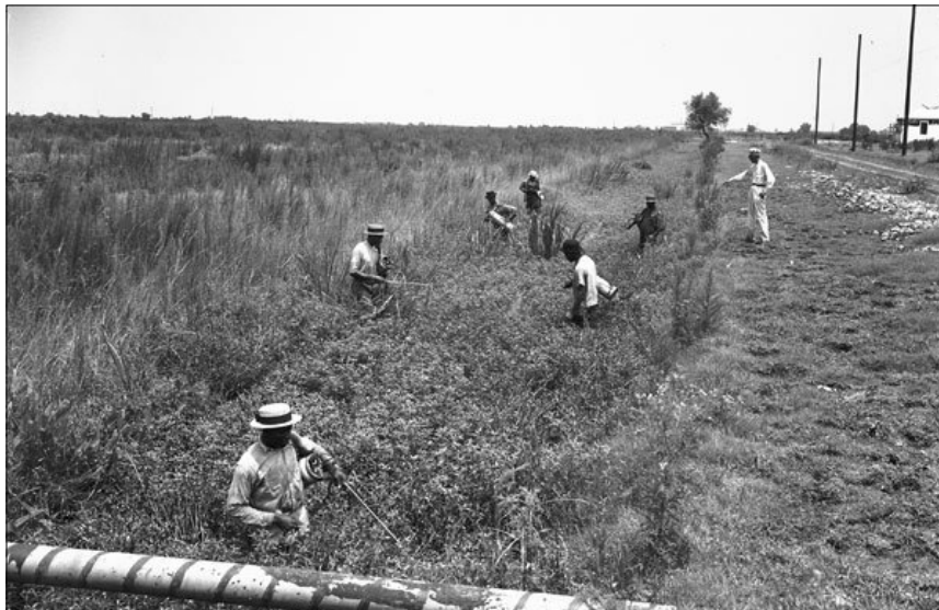
Photographs showing the Works Progress Administration's early efforts at mosquito control capture how methods have changed over the decades. In this photograph, taken in 1941, WPA workers in Louisiana are spraying fuel oil in a ditch. (Photograph: WPA archive, http://nutrias.org/photos/wpa/images/35/350210.jpg .)
