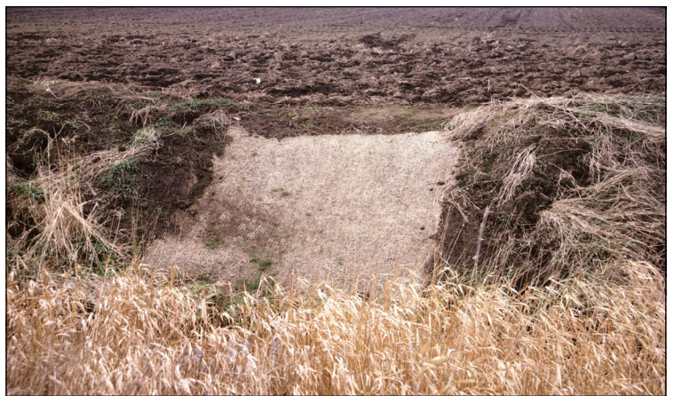
Geotextile reinforced grass chute
