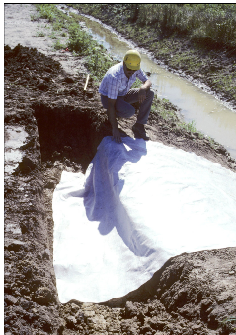
Laying out geotextile for grass chute
