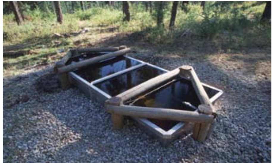
Soil stabilization is critical around water troughs.
