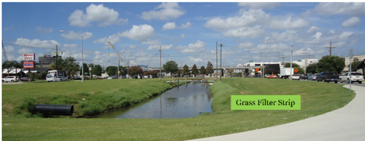
Figure 5-12: Grass filter strip along Veterans Highway north of Causeway Boulevard
