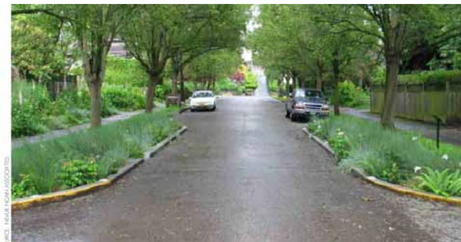
Figure 5-7: Curb extensions retrofitted into a residential street (San Mateo 2009)
