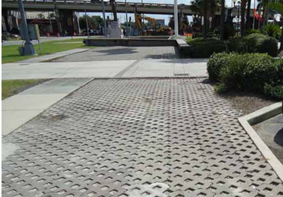
Figure 5-4: Permeable pavers at the Lakeside Mall (Jefferson Parish)
