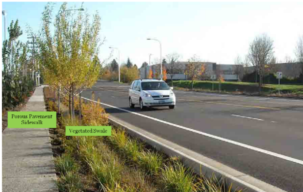
Figure 5-11: Arterial roadway with vegetated swale and porous pavement sidewalk (modified from San Mateo 2009)
