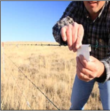
Figure 2. Installation of a fence marker.
