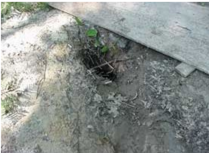
Abandoned wells are pathways for contamination of the groundwater.
