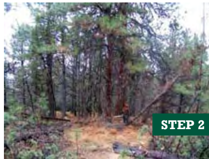
Step 2 – removing small diameter trees
