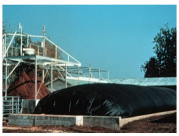
An operational anaerobic digester
