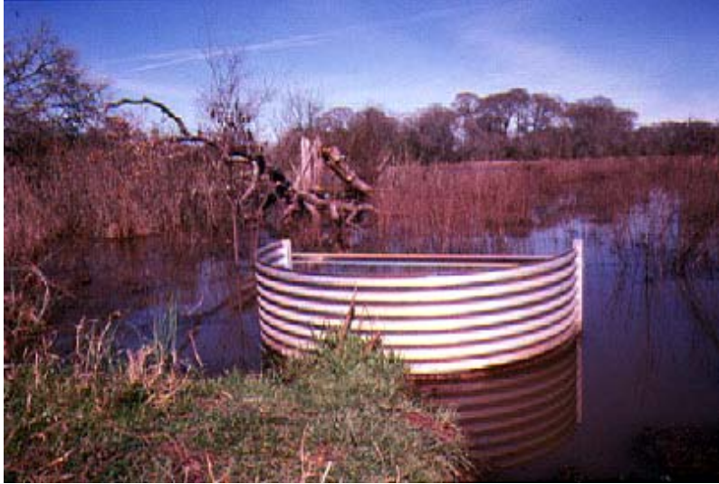
A water control structure built into a levee can create a shallow wetland that will benefit waterfowl and other wetland species.
