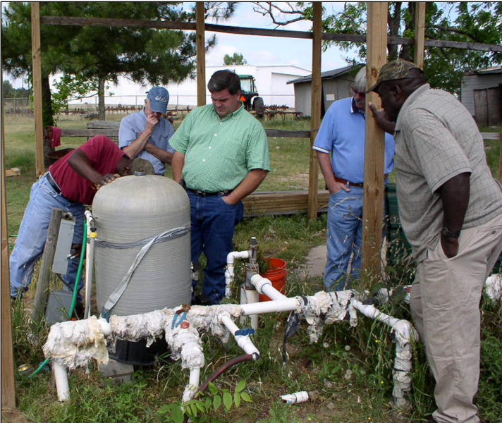
Dividing solid set irrigation systems into smaller zones can be accomplished by use of an irrigation manifold
