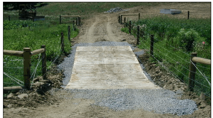
Hog panel stream crossing
