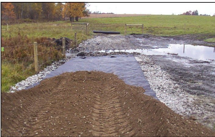
Stream crossing under construction
