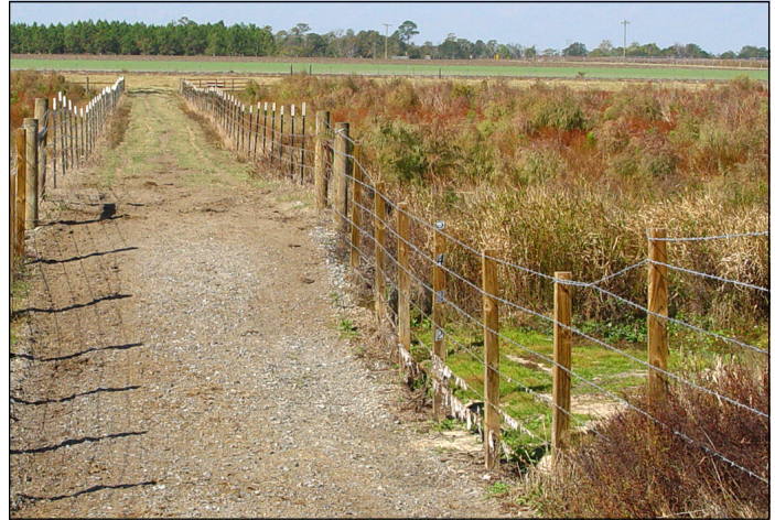
Fencing restricts livestock access to the crossing and protects the stream
