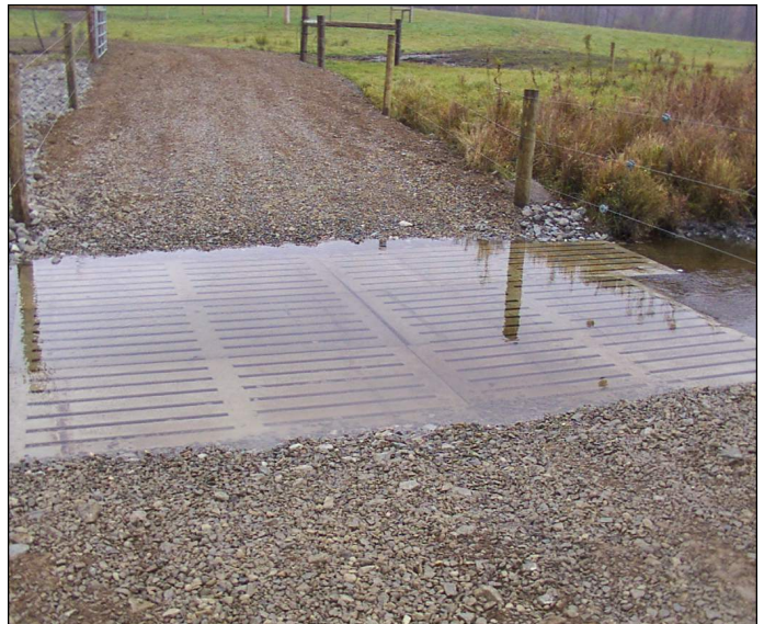
Hog panel stream crossing
