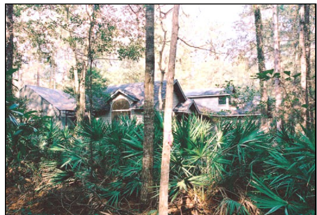
Property surrounded by highly volatile vegetation increases its vulnerability to wildfire.
