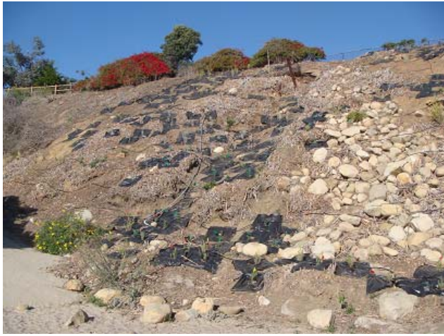
Figures 25 and 26. Plants were planted through ground cloth to discourage weeds, erosion, and conserve water. Squares were used to keep costs down. Irrigation was provided for each plant.
