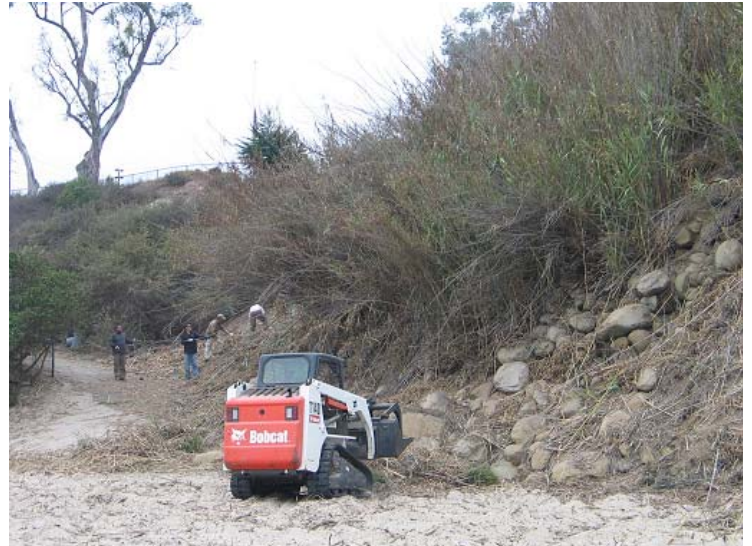
Figure 9. Primary removal of large middle patch at end of sidewalk
