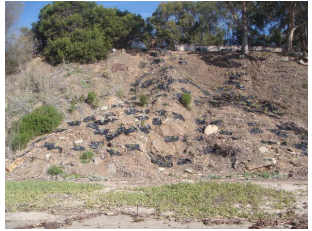
Figures 25 and 26. Plants were planted through ground cloth to discourage weeds, erosion, and conserve water. Squares were used to keep costs down. Irrigation was provided for each plant.
